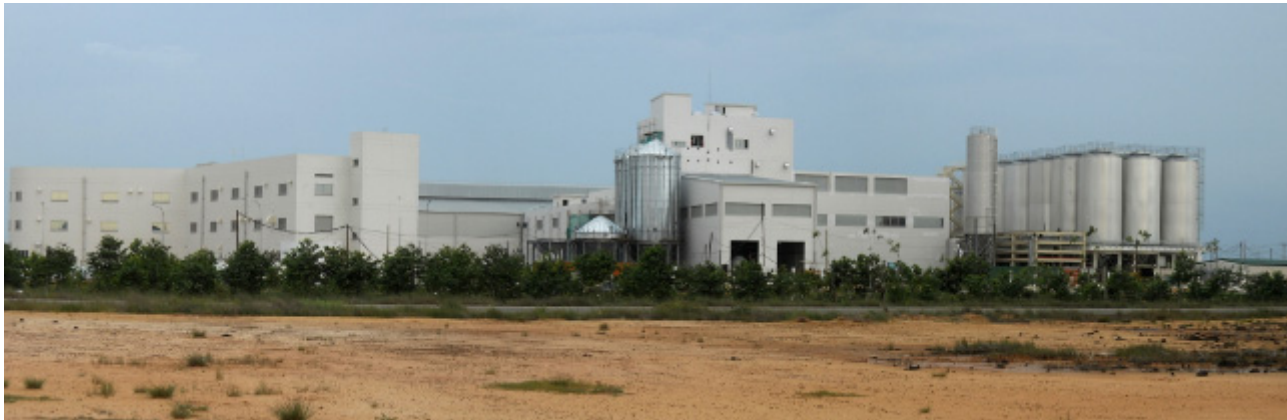
Vietnam plant under construction (June 29)
